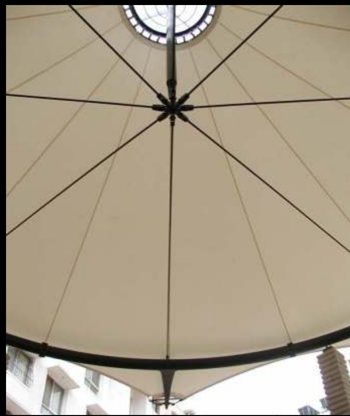
CENTRAL JOINT WITH SKYLIGHT
